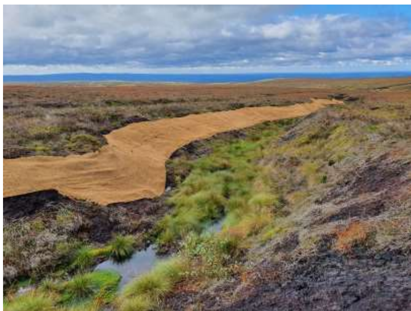
Geo-textile laid to protect the gully side, ready for seeding & brash; revegetation on site 2 years after the original work
